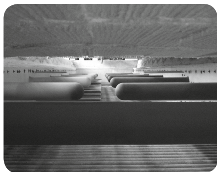
Ceramic radiant tubes SER-C in roller hearth furnace during installation work
