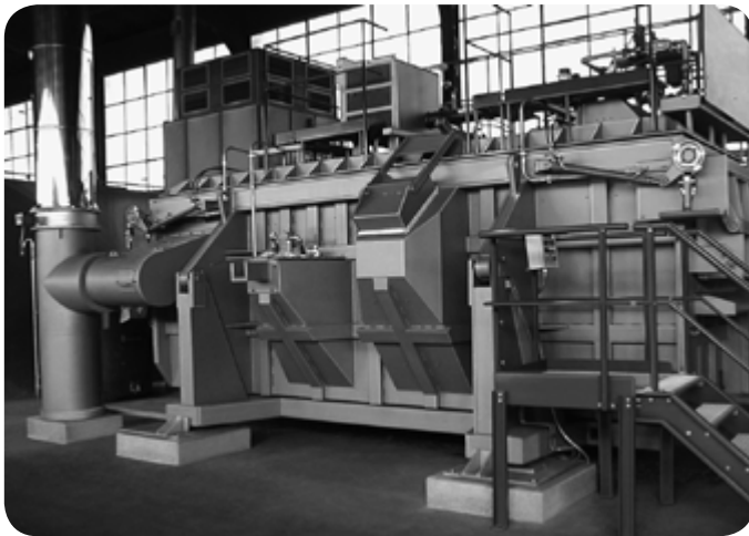
Aluminium industry: smelting furnace
